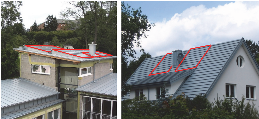
Figure 6-1 Two Systems with roof integrated uncovered zinc collector marked in red. Left: System in Limburg with 44 \text{ m}^2 collector area; Right: Klein Köris System with 20 \text{ m}^2 collector area
