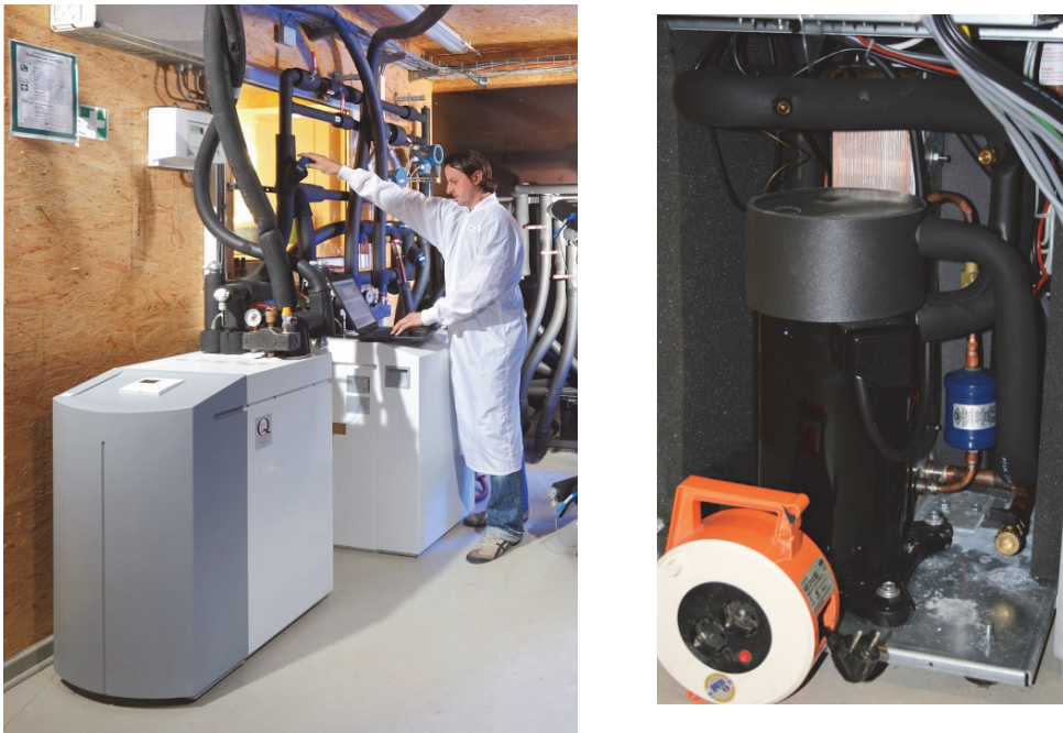
Figure 2-1: Left: Compression heat pump at test facility at ISFH. Right: Glance into the inner parts of the heat pump: Black cylinder-compressor, silvery box behind the compressor-plate heat exchanger
