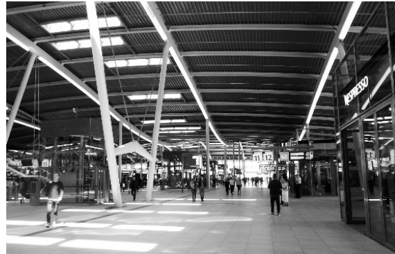
Figure 72 Side and inside passage of the station. Source: author, 2017.
