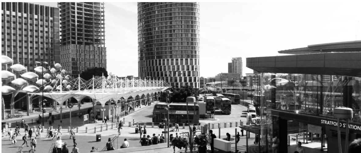
Image 57 Stratford Station area and surrounding residential buildings. Source: Author, 2016.
