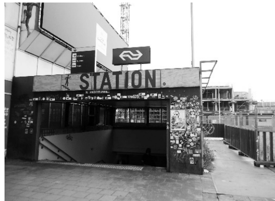
Figure 70 North tunnel [Nooertunnel]. Element of connection and direct access to the platforms of shipment. Source: author, 2017.
