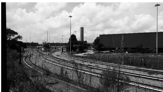
Shed for the maintenance of the trains in the Maneuveryard in the northern sector.
