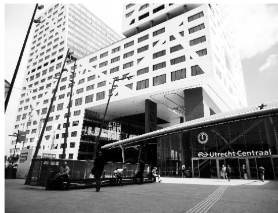
Figure 108 West facade of the Central Station, partially prefecture building on the entrance and lateral access connec- tion between the banks. Source: author, 2016.
