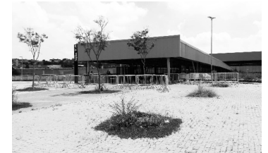
South facade of access to Itaquerá subway and train station.
