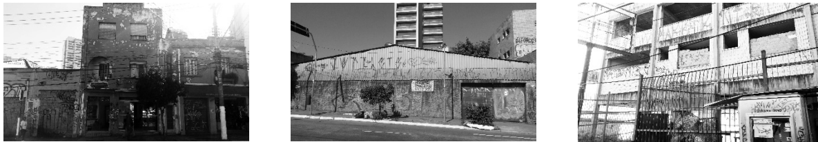
Figure 13 Buildings deteriorated and/or for sale in the Faria Lima station area. Source: author, 2017.
