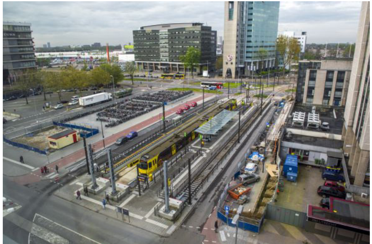
Figure 48 Temporary terminal of trams and buses while the works of the surroundings are not finished. Source: CU2030, 2017.
