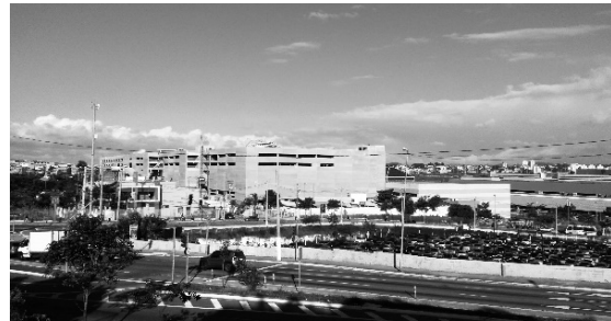
North facade of the mall and its expansion in 2017.
