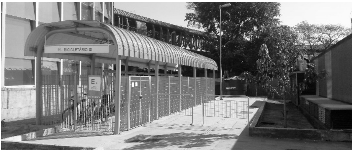
Figure 45 SPTrans Bicycle Racks - between station and terminal. Source: author, 2017.
