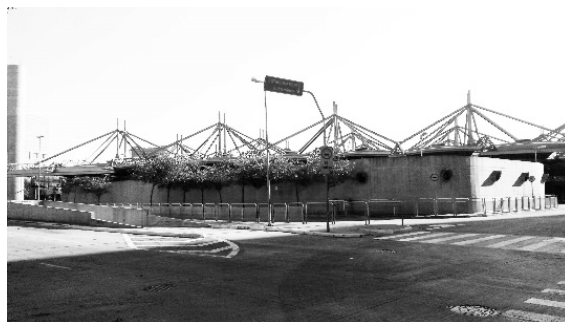
Figure 79 South facade and east of the terminal respectively in the street Capri. Source: author, 2017.
