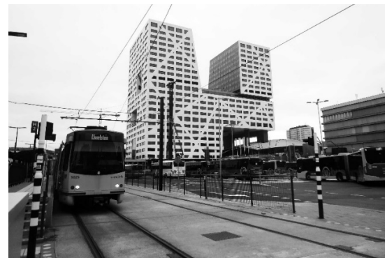
Figure 88 Tram terminal next to the bus terminal and access to the station - Jaarbeursplein Square (temporary). And access street adjacent to the tram terminal. Source: author, 2016.
