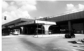
South facade of the subway station adjacent to East Radial Avenue along with the facade of the bus terminal.
