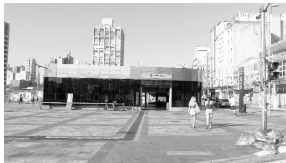
Figure 78 West facade Faria Lima Station (exit Largo Batata) and exit Teodoro respectively. Source: author, 2017.
