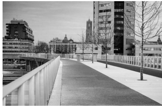
Figure 71 Rail pass on Moreelsebrug . Source: CU2030, 2017.
