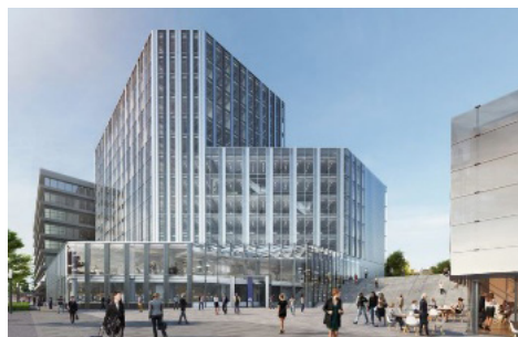
Figure 54 Knoopoffices - Node of offices for public sector) Source: CU2030, 2017.
