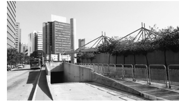
Figure 29 Sidewalk immediately in front of the bus terminal (Gilberto Sabino street). Source: author, 2017.
