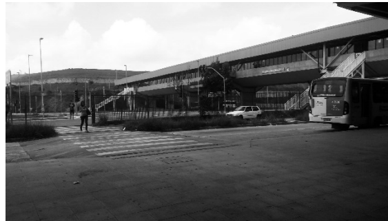
Figure 45 Bus stop heading downtown and bay for landing / boarding on the avenue. Radial Leste; gate access to the bus terminal on Avenida Radial Leste. Source: author, 2017.
