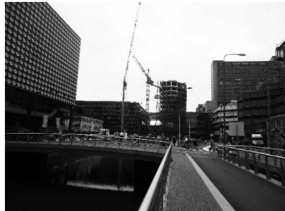
Figure 77 Current cycle path on the street Vredenburg and the bridge for pedestrians and cyclists ( Vredenburgknoop ) Source: author, 2016.
