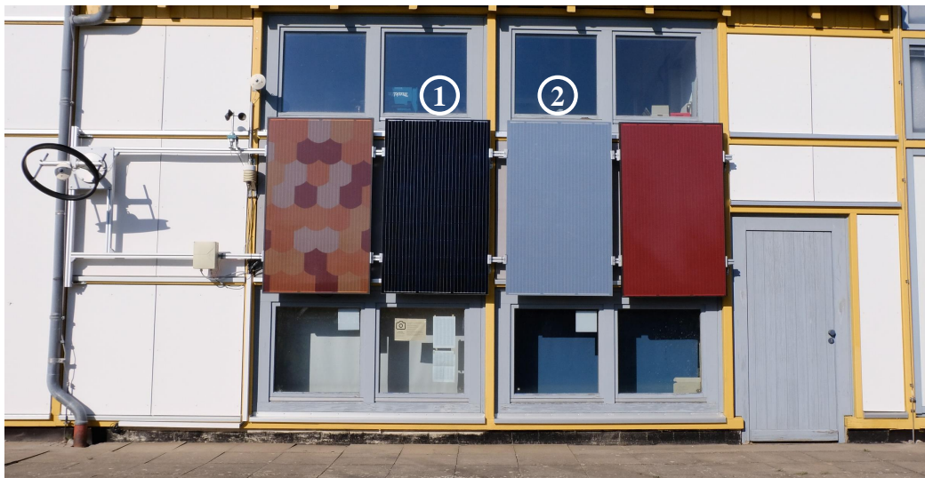
Figure 4.22: Standard PV module (1) and a greyish CoTex module (2) on a façade.
