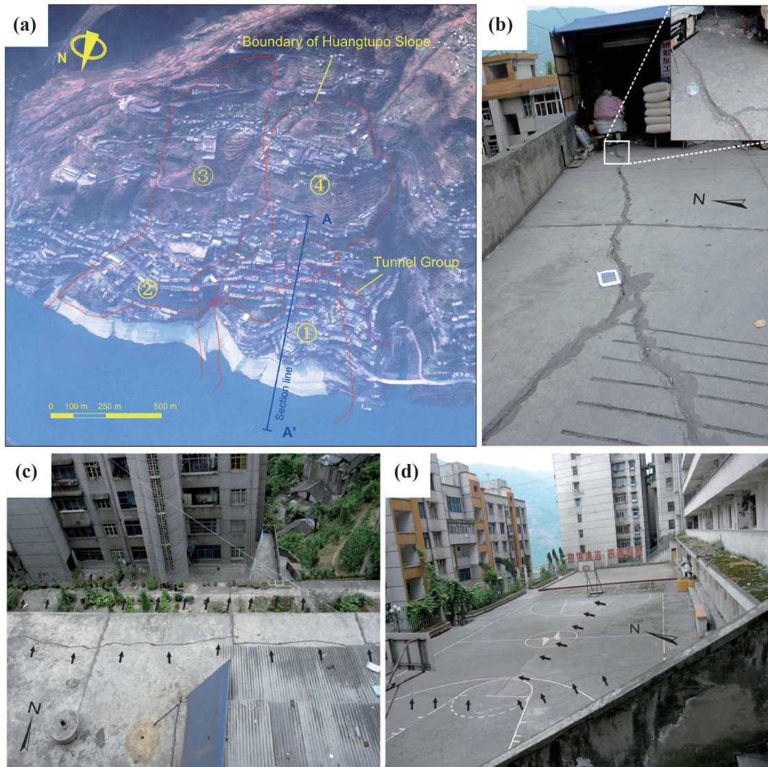
Figure 2.6: (a) Example for one of the largest slow-moving landslides in China, i.e., the Huangtupo landslide, with annual displacement rates of around 10–20 mm/year. (b) Examples of the potential damages for the slow-moving Huangtupo landslides. Note that north arrows approximately indicate the downhill direction. (Source: adapted by Wang et al. (2018) and Tomás et al. (2014).)
