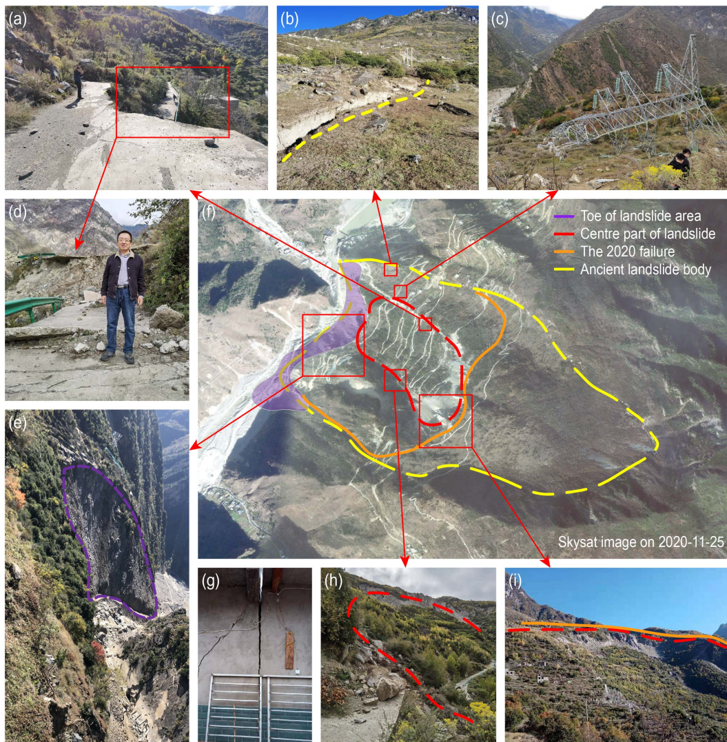
Figure 4.2: Display of the landslide failure and different zones of the landslide body, as well as examples of damages in the event. (a) Ravaged roads on the edge of the central failure. (b) The northern lateral flank of the landslide. (c) Damaged extra high voltage (EHV) transmission tower. (d) Front view of ravaged roads. (e) The toe of the landslide body. (f) Skysat optical image acquired on 25 November 2020, with the boundaries of three different zones of the landslide, i.e. the red, orange and yellow lines represent the areas with the fast, medium and slow movements in this event, respectively. (g) Cracked house. (h) The southern flank of the center part, which had the fastest displacement rates during this failure. (i) The main scarp of the failure in the southeast direction.
