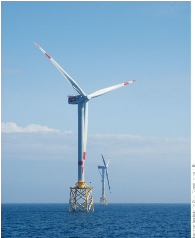
Fig. 4 Jacket in the Alpha Ventus wind farm
