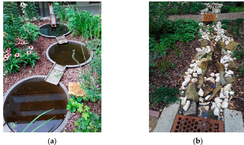
Figure A2. (a) One of the cistern cascades in the courtyard. (b) Channel to one of the ponds in the courtyard.
