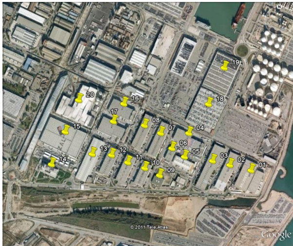
Figure 7. Selected buildings on industrial area of Barcelona
